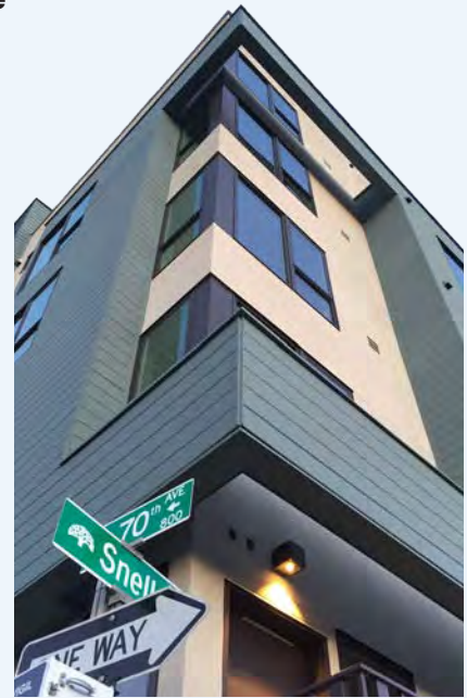
Intensive planning helped achieve goals like a shorter construction schedule for Coliseum Connections.
