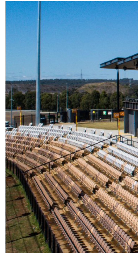
Sydney International Speedway. Built by Fleetwood Australia. Winner, Permanent Special Application Over 10,000 Sq. Ft.
