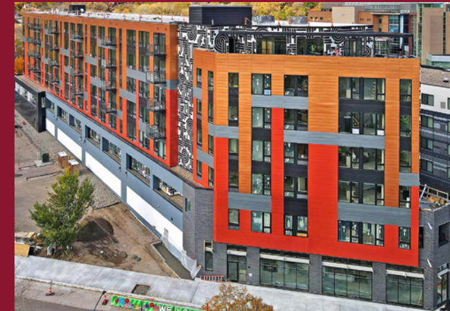
Cover Image: Alvera Apartments. Built by RISE Modular. Winner, Permanent Multifamily Over 10,000 Sq. Ft.
