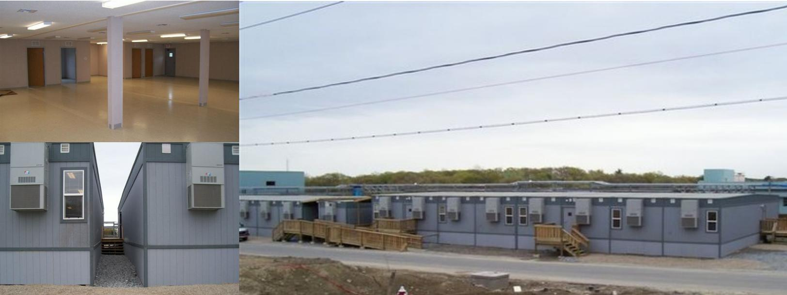
The site at Devens has required a combination of modular units to provide temporary space to support the Bristol Myers Squibb's manufacturing facility construction project. Triumph Modular has supplied more than 36,400 sq ft of modular space for office, conference, orientation, safety, and bathroom facilities.
