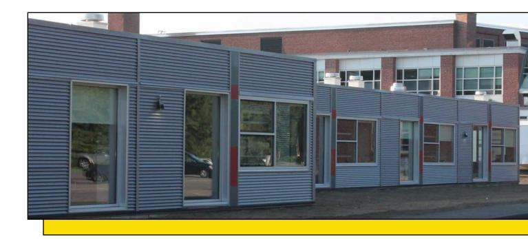
Triumph Modular provided Lexington High School with 18,000 sq. ft. of classroom space over the summer break. The building was ready for the first day of school, on time, and within budget. The building features a high efficiency HVAC system, corrugated steel siding on the exterior, and expansive floor-to-ceiling glass, which allows the classrooms to be illuminated with natural light.
